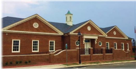
The newly renovated Juvenile and Domestic Relation Court opened in September of 2015.
