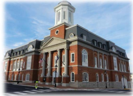
The Fredericksburg Courthouse houses the Circuit Court and the General District Court. It opened in August of 2014.
