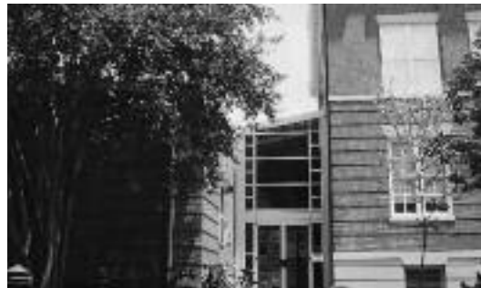
Central Rappahannock Regional Library Annex, Fredericksburg
