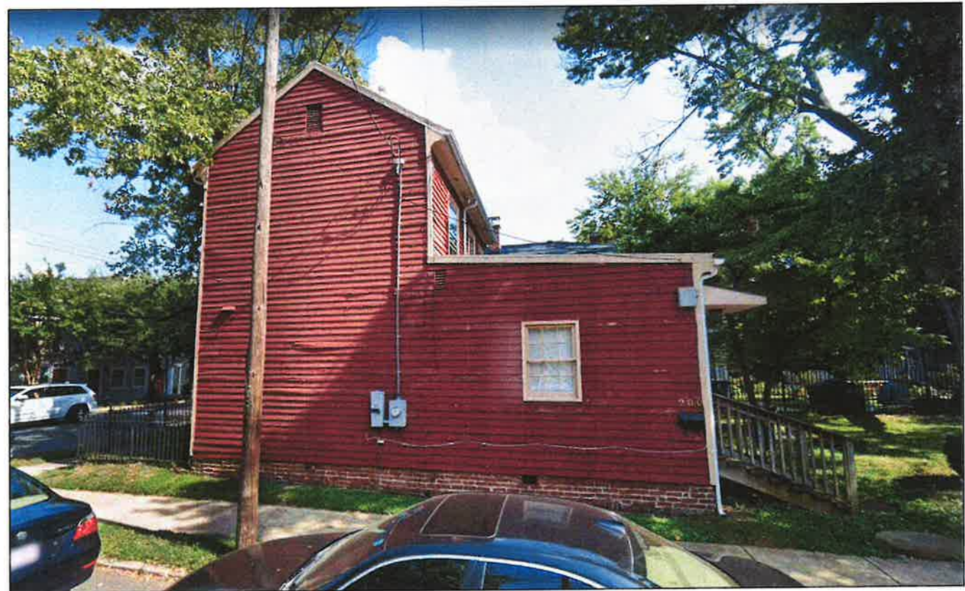
○ PHOTO OF EXISTING STRUCTURE FROM NORTH
