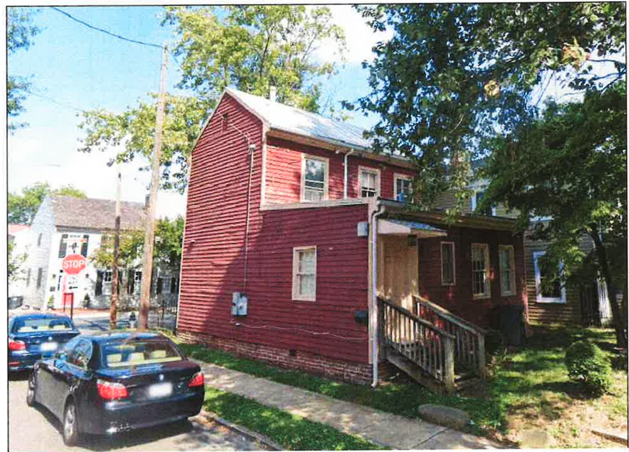
○ PHOTO OF EXISTING STRUCTURE FROM NORTH
