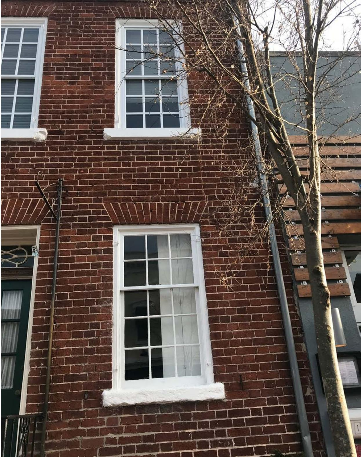
Replacement vinyl sash shown on the second floor; existing wood windows on the first floor. The second floor and dormer windows will be replaced with custom wood windows that match the details of the first floor.
