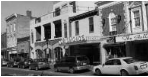
900 Block Caroline Street, Fredericksburg
