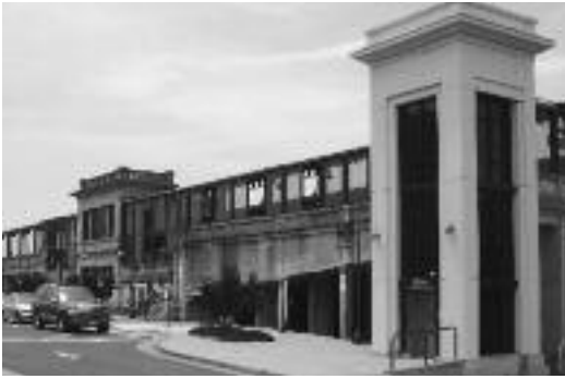
Railway Station, Fredericksburg
