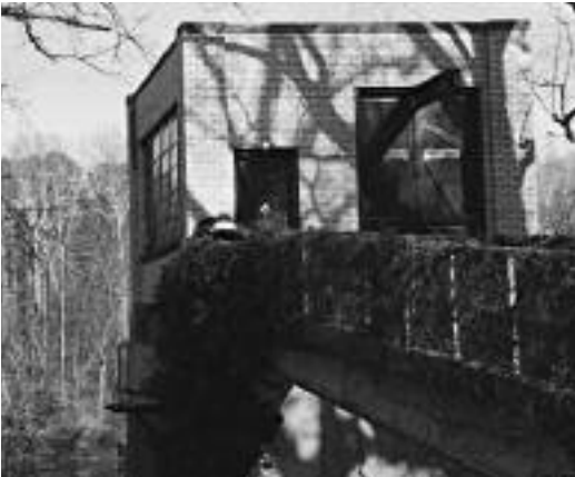
Pump Station, Fredericksburg
