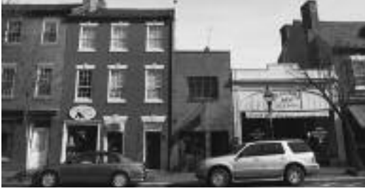
700 Block Caroline Street, Fredericksburg
