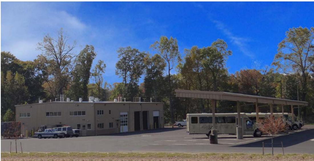
The Maintenance building has an in-ground heavy duty lift and a mobile automated lift system, a wash bay, a fueling station, and covered bus parking. These features will
